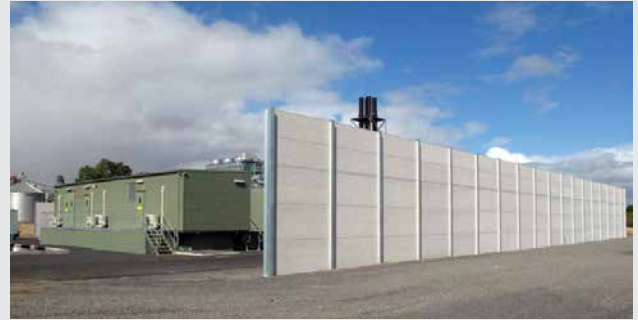
Acoustic Wall Barrier to power station
